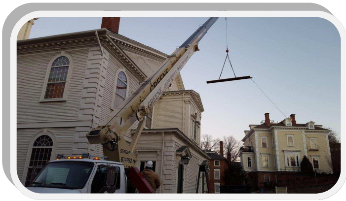
At about 7 a.m. on Friday, January 22, a crane arrived and hoisted the beam up where it could be brought into the attic area of the
